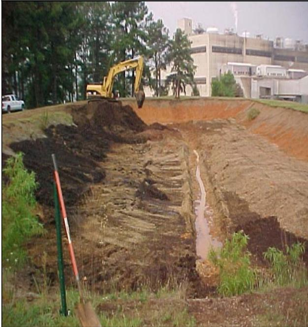
Georgia Power Company required the removal of sediment from two unlined Boiler Cleaning Waste Basins (BCWB's) at their Plant Yates facility. Following the removal all sediments, a 60-mil HDPE liner needed to be installed prior to the plant's scheduled boiler maintenance activity. SBX Technologies, LLC was awarded the contract based past BCWB experience, excellent safety record and the ability to meet the time-critical schedule for the work.
