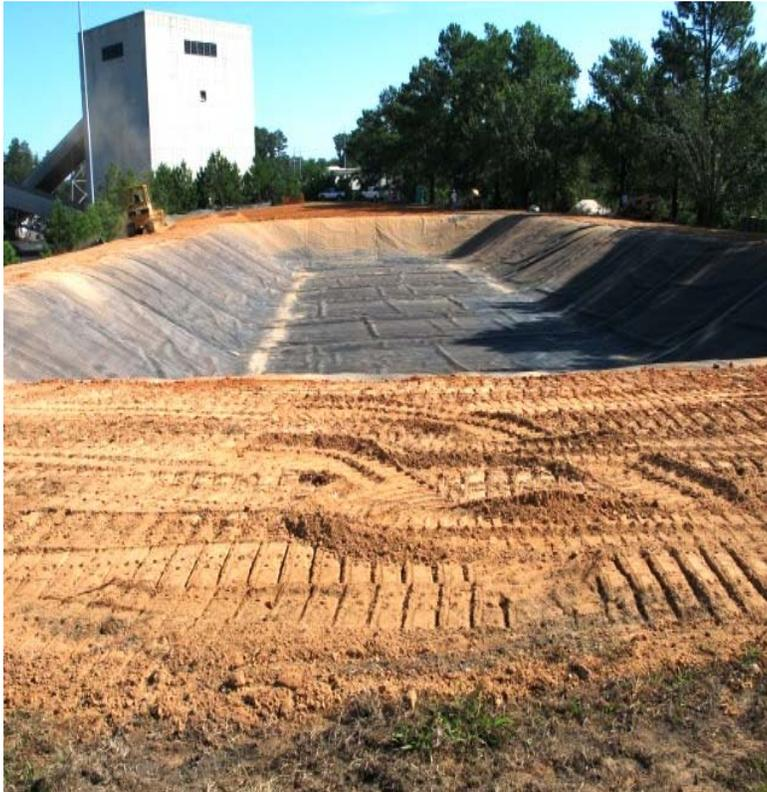
The liner trench was backfilled and compacted in 6-inch lifts during the morning to minimize the liner lifting from the bottom of the basin during cool periods. Following the completion of the liner installation in the large basin, all disturbed areas were graded to the final elevations and contours then seeded.
