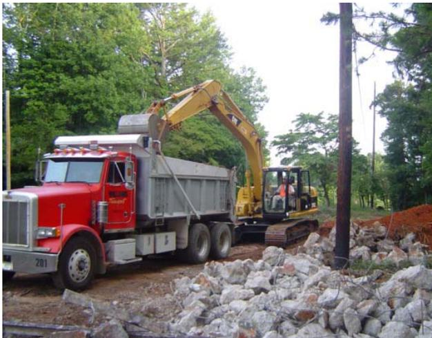
**Excavation quantities typically range from a few hundred to a few thousand tons of impacted soil and concrete and are transported to a licensed landfill facility. After the impacted soil areas are excavated, a specific sampling grid is measured out and confirmation soil samples are collected and analyzed. When analytical results are below acceptable levels, SBX imports acceptable fill material to backfill the excavated areas. The sites are seeded and fertilized to control erosion.**
