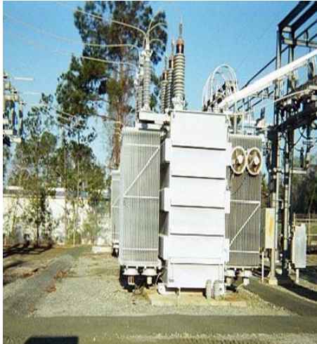
Rock containment berm
