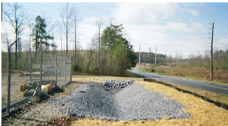
Oil detention pond
