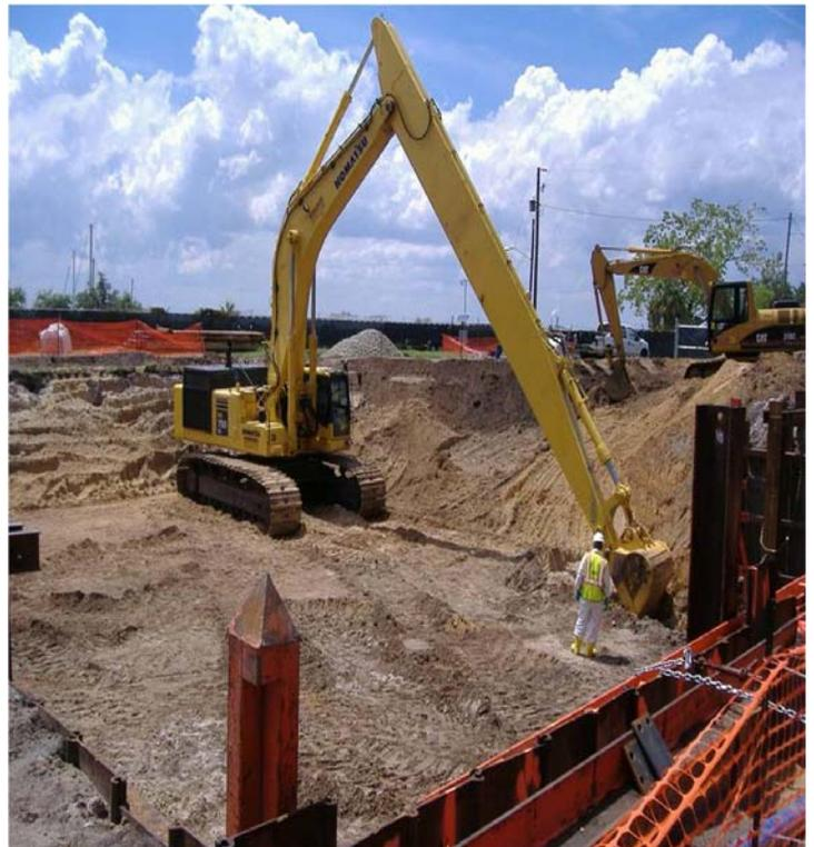
The SEA utilized a Portland Cement/Bentonite slurry to displace excavated soil and would remain in place as saturated zone backfill. The slurry was designed to exhibit clay-like physical characteristics after curing. The saturated zone soil was excavated using a 75-ton excavator with a long-stick attachment and a 5-foot wide bucket. A batch mixing plant was used to mix the slurry and a grout pump was used to deliver the slurry to the excavation area.
