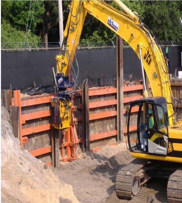
The Former Brunswick Manufactured Gas Plant (MGP) represented the major challenge of removing source material from the saturated zone. Previous Removal Actions had excavated source material from the unsaturated zone down to the groundwater elevation, a depth of approximately 14-feet below ground surface (BGS). To further complicate the project, the site had a limited footprint of less than one acre and was situated less than 100 yards from the bay in Brunswick, Georgia.
