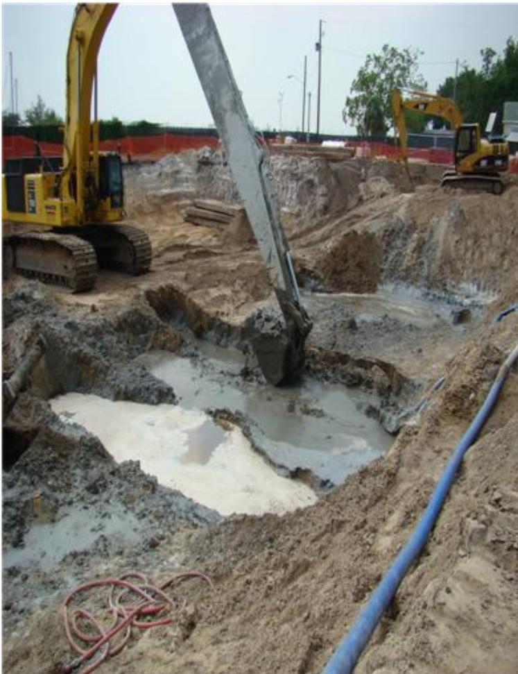
The excavated material was placed on a curbed concrete pad to allow water to drain from the saturated soils. This water, along with any decontamination water was treated by the on-site water treatment plant, and then reused in the slurry batch plant. After dewatering, the soils were stockpiled on the concrete pad and scheduled for loading and off-site disposal.
